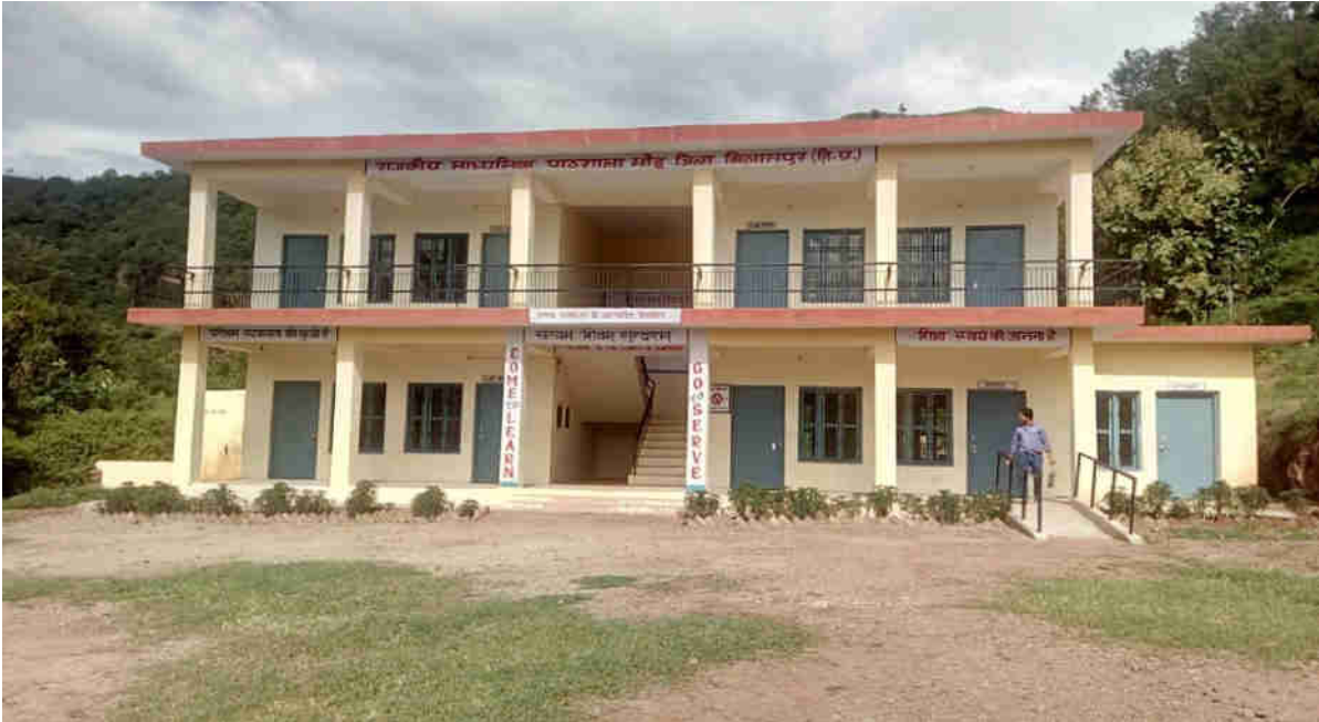
New Upper Primary School Building at GMS, Mohru, District Bilaspur (HP)
