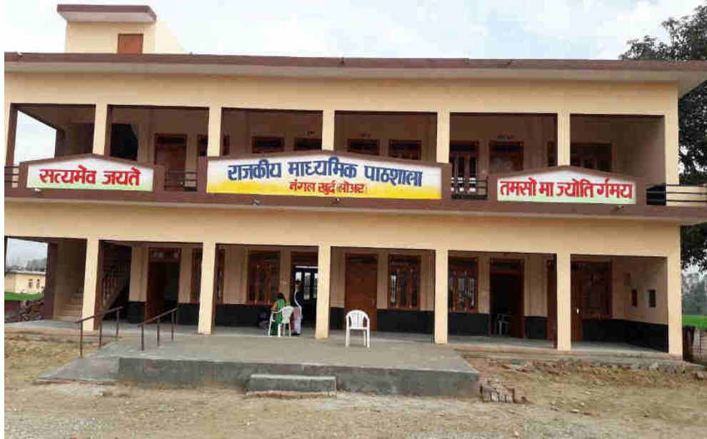
New Upper Primary School Building at GMS, Nangel Khurd, District Una (HP)
