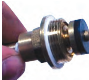
Fig. 5.8: Replacing the rubber washer
