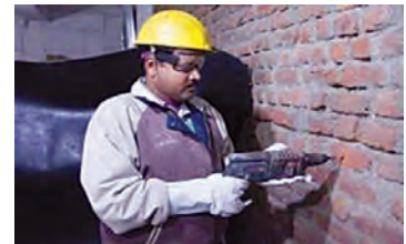
Fig. 6.1: Using power drill machine
