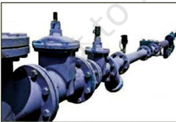
Fig. 5.27: Flanged joints
